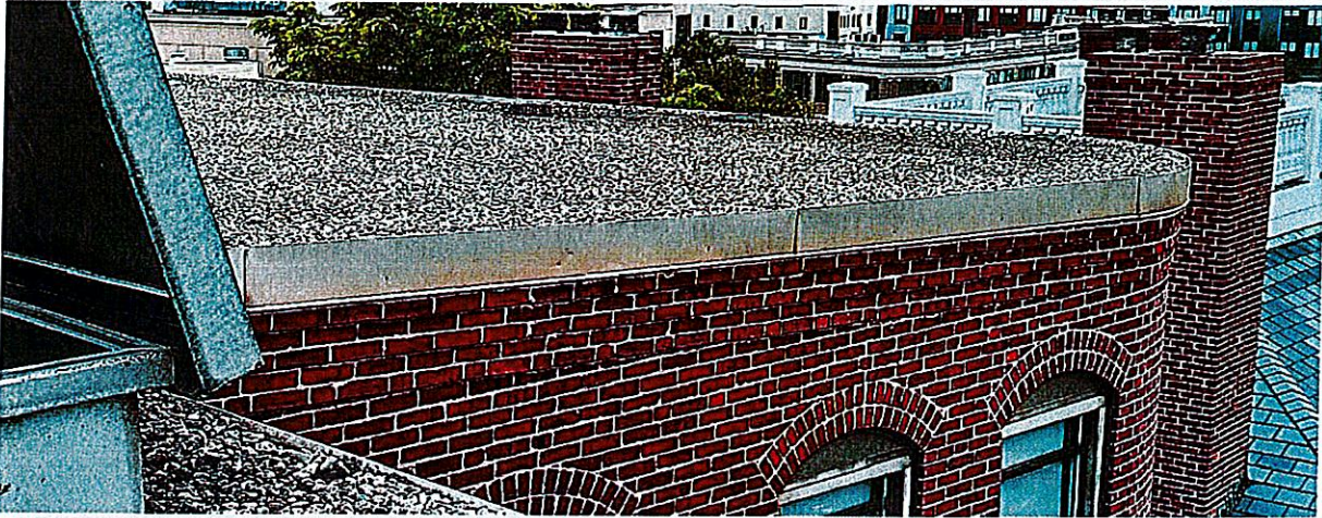
Brick cornice before construction
